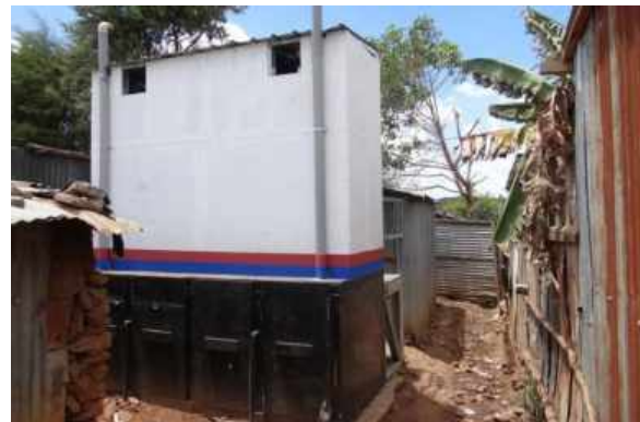
Figure 8: Open urine pipes
