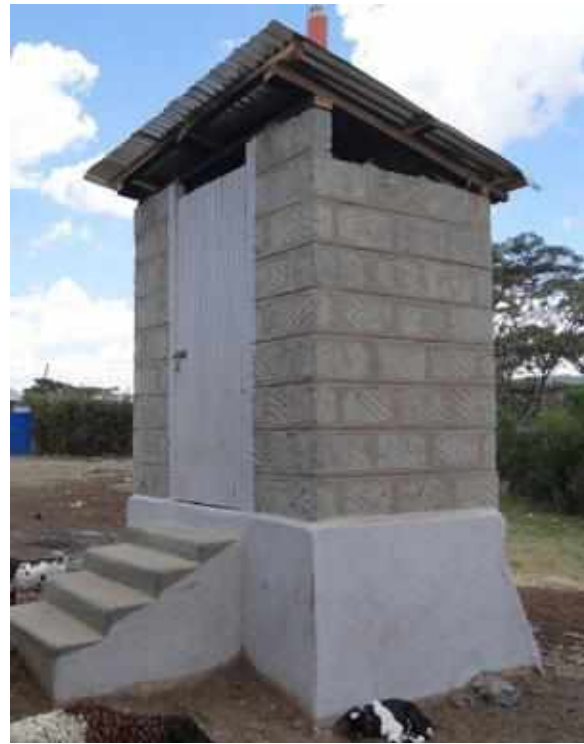
Figure 1 – SafiSan in-situ build toilet
